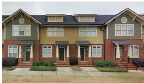
Multiplex Small 105 S. Memminger Street 4 units in building, 1 in each Townhouse; resultant density: 30 du/ac
