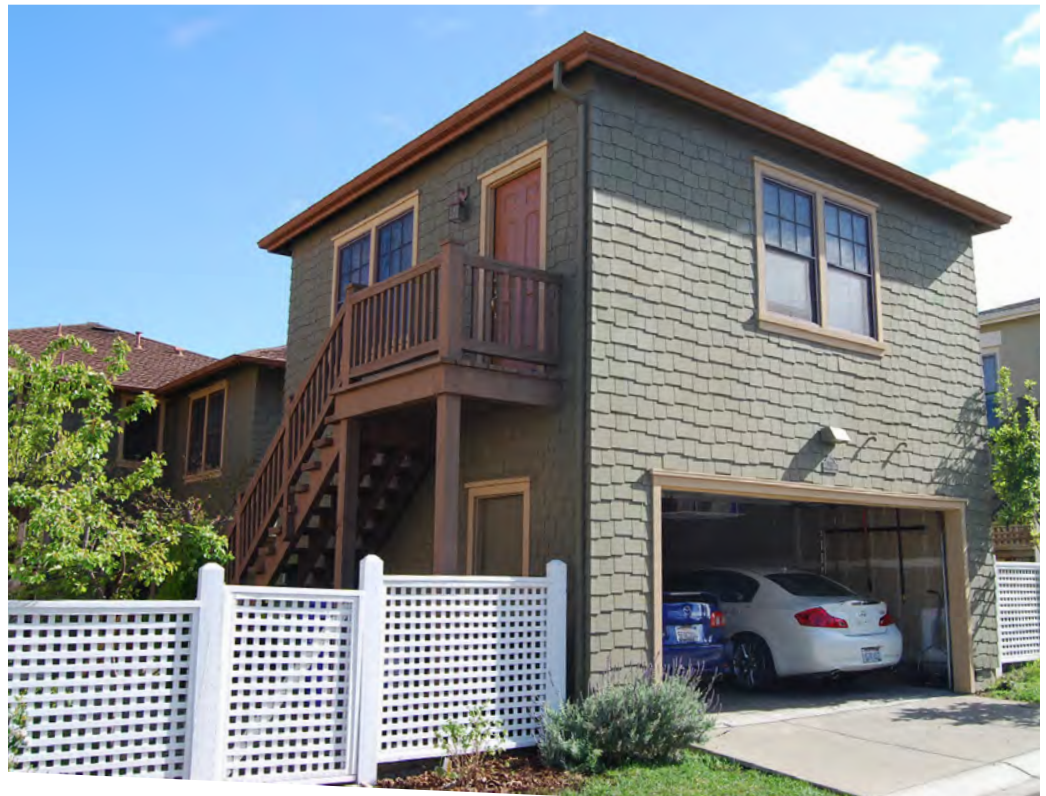
An ADU can be on top of a garage or at grade near or attached to the garage, but always is smaller than the primary building on the lot. This ADU contains approximately 600 sq. ft..
