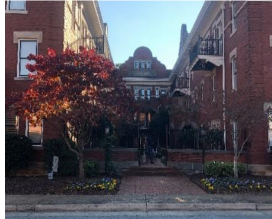
The Davenport was built in the 1900's and is part of a district that provides a transition from dense urban core (downtown Greenville) to surrounding neighborhoods.
